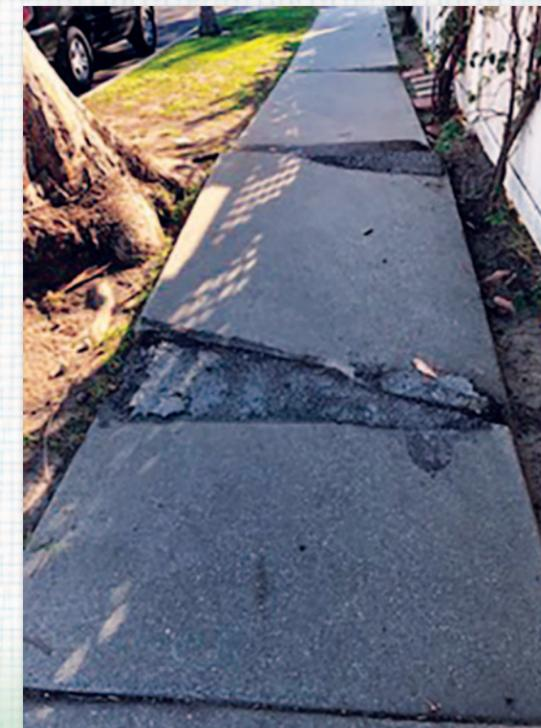
Broken sidewalk caused by street (city) tree
