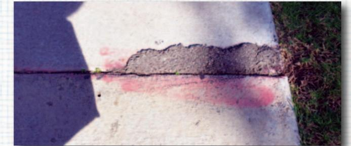
uplifted sidewalk. The city may also fill in cracks rather than replace it.
